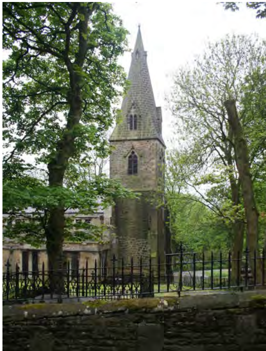
The 1854 church tower and spire by Hadfield and Weightman. (Tower and Spire of All Saints, The Builder, 16 Sep 1854, p.489)
